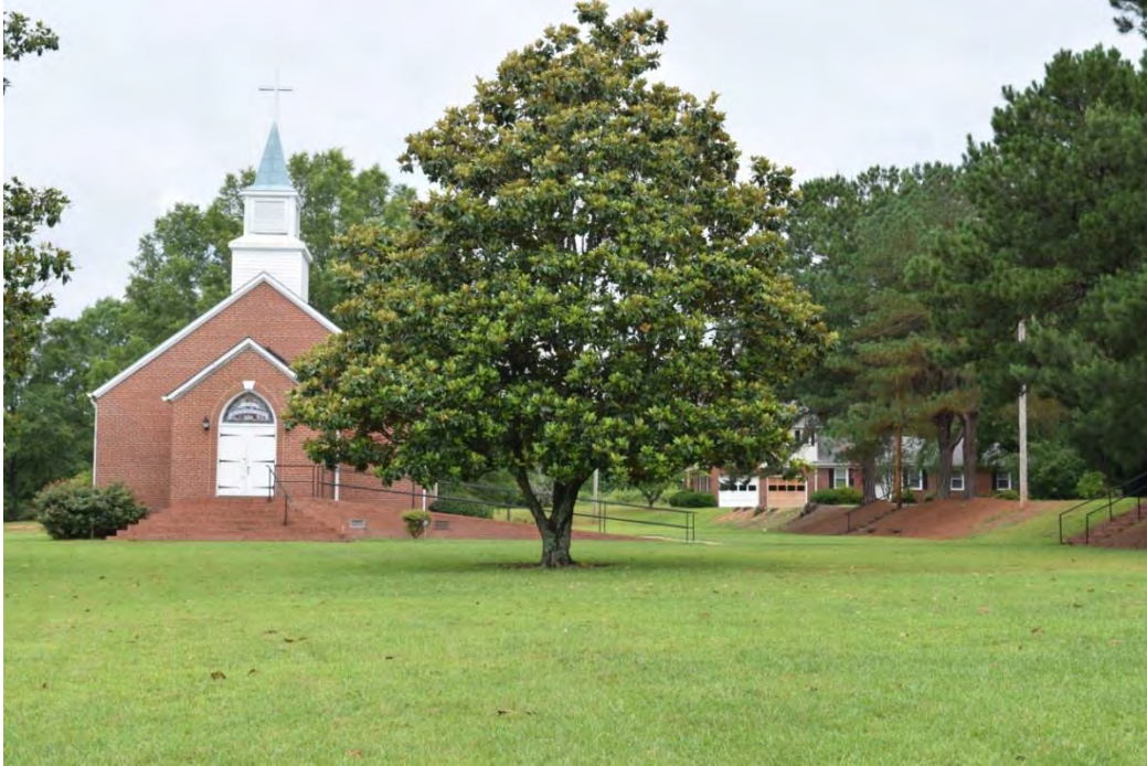
Wade Manufacturing Company Mill and Mill Village Historic District, Wade Methodist Church and Parsonage, Looking West.
