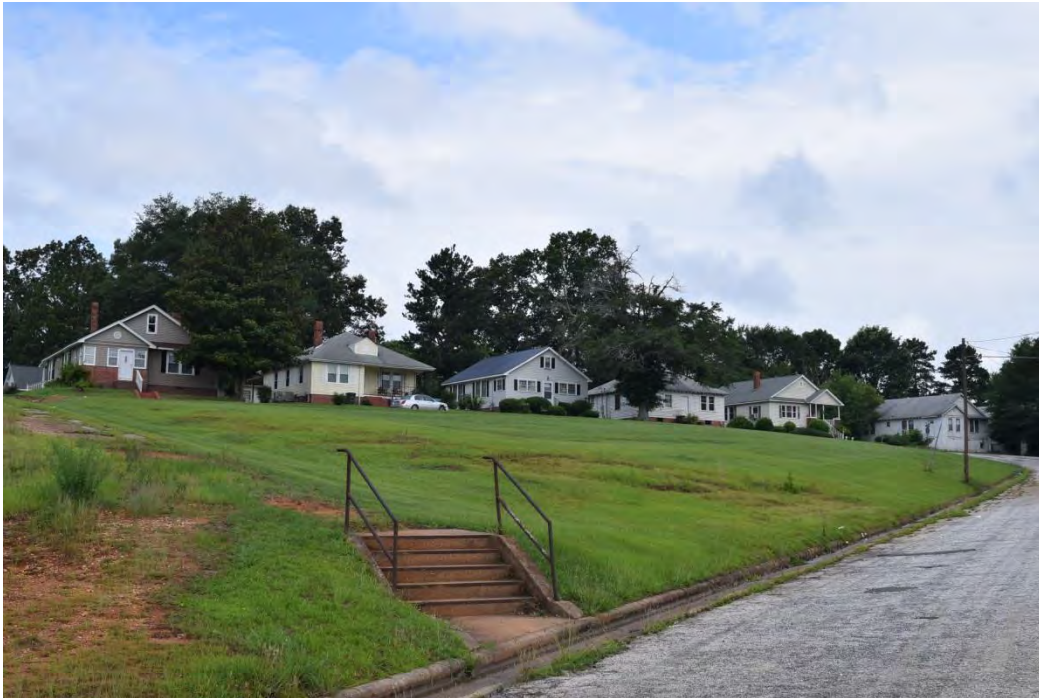
Wade Manufacturing Company and Mill Village Historic District, Mill Village, Looking Northwest.
