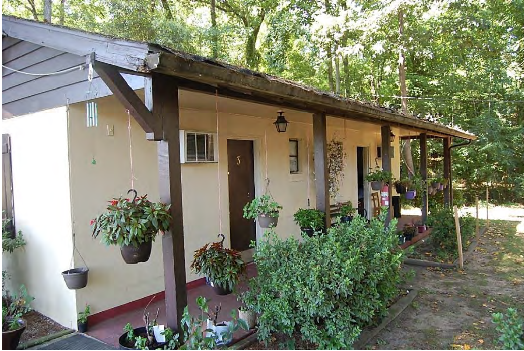
Valley Motor Court, South Building, Looking West.
