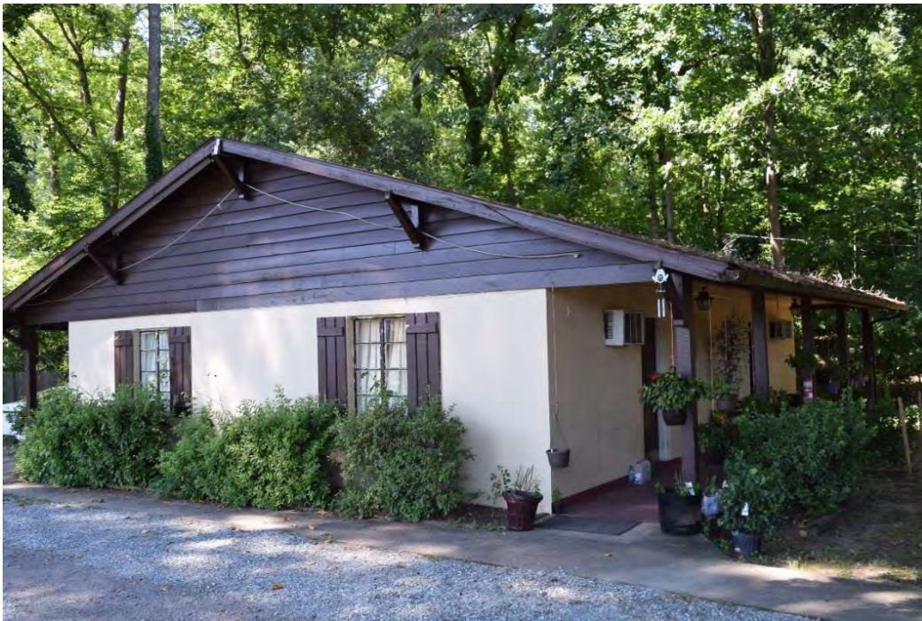
Valley Motor Court, South Building, Looking West.
