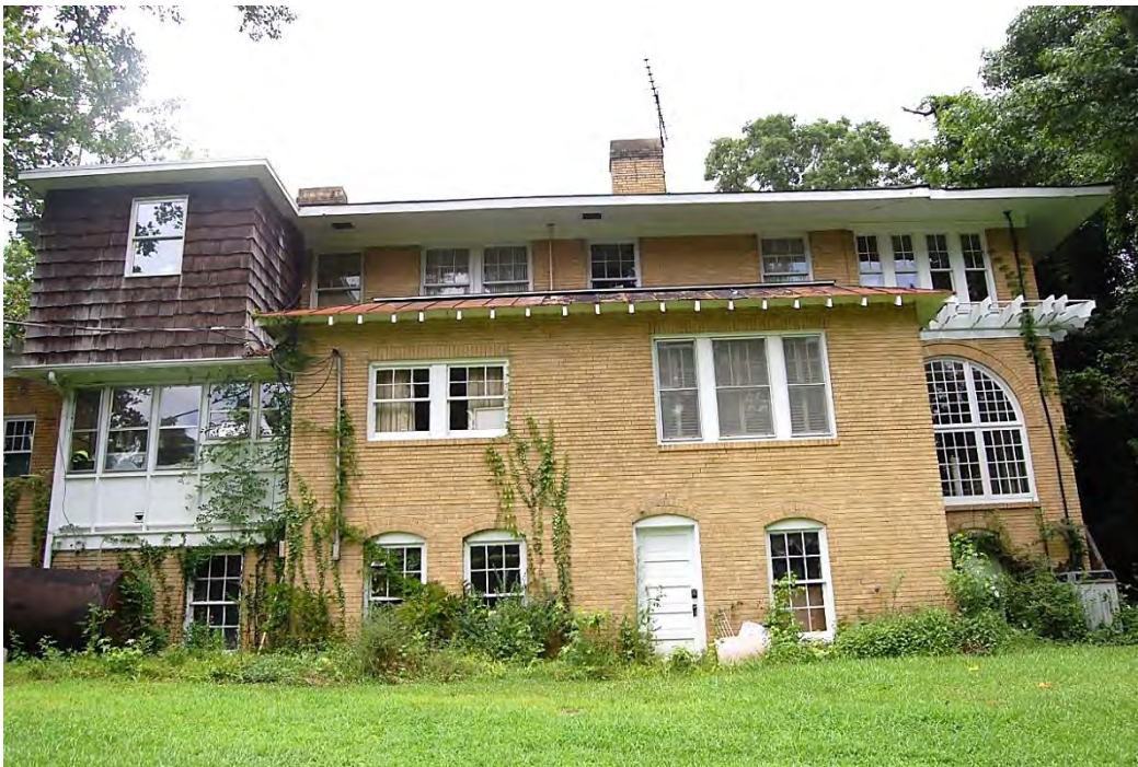
Caudle Family House, Rear (South) Elevation, Looking North.
