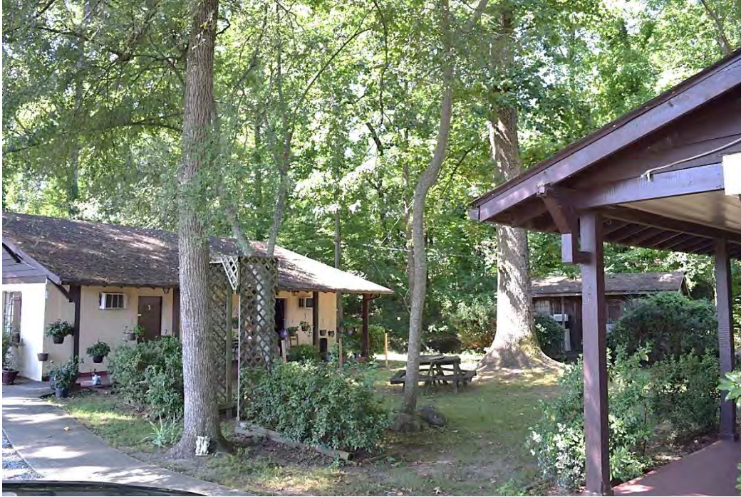
Valley Motor Court, Courtyard between Office Building (Right) and South Building (Left). Modern Prefabricated Storage Building to the Rear, Looking Southwest.
