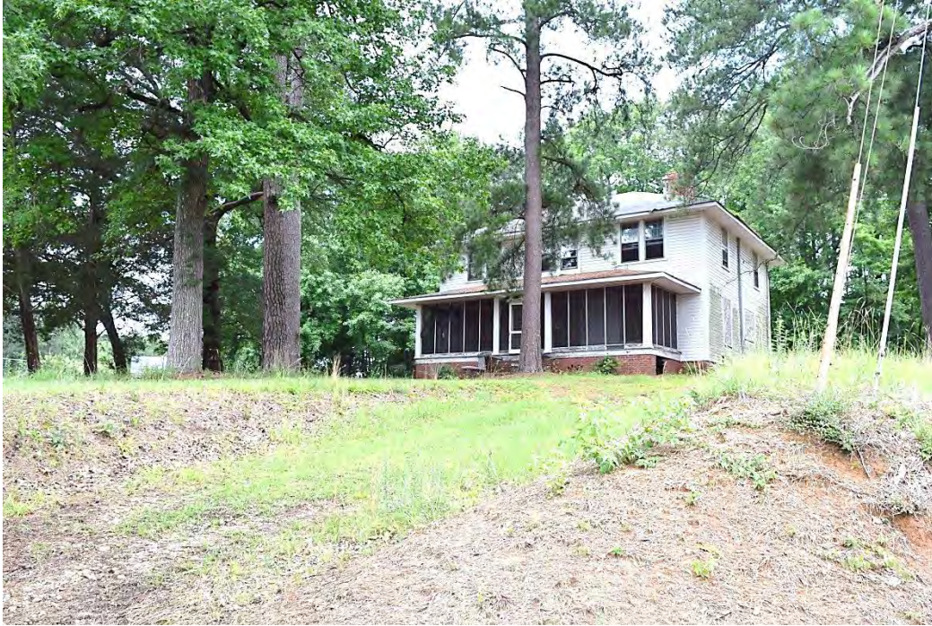
Wade Manufacturing Company and Mill Village Historic District, Mill Superintendent's House, Looking North.
