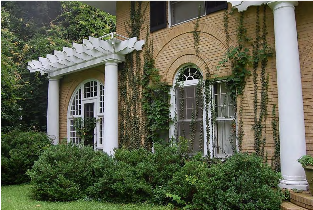
Caudle Family House, Facade, Windows and Sunroom, Looking East.
