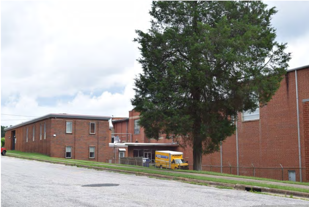
Wade Manufacturing Company and Mill Village Historic District, Original 1923 Mill, Postwar Addition in Right Foreground, and Postwar Office Building, Looking North.
