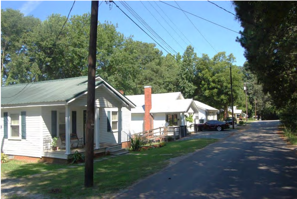
Wadesboro Cotton Mill Village, ca. 1950 Houses at 204-206 Hargrave Street, Wadesboro.
