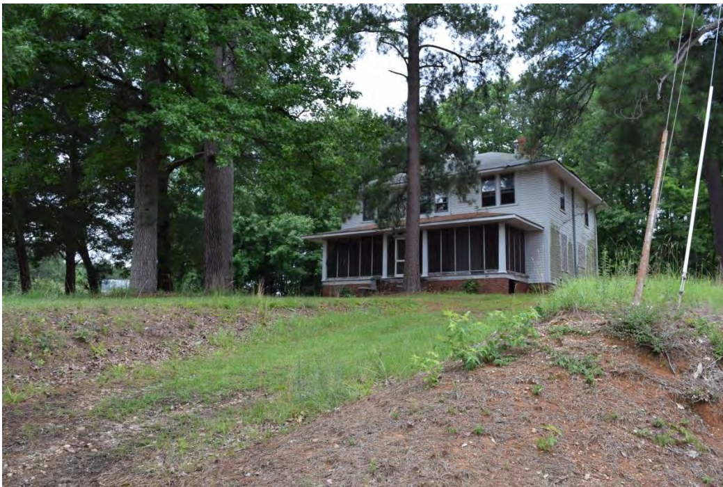
Wade Manufacturing Company and Mill Village Historic District, Mill Superintendent's House, Looking North.
