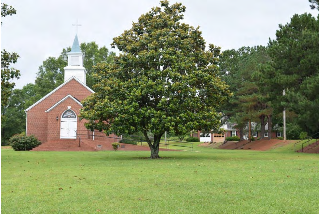
Wade Manufacturing Company and Mill Village Historic District, Methodist Church and Parsonage, Looking West From Church Street.
