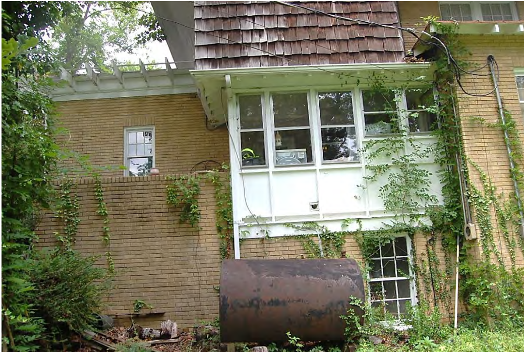
Caudle Family House, Rear (South) Elevation, Utility Porch, Looking North.
