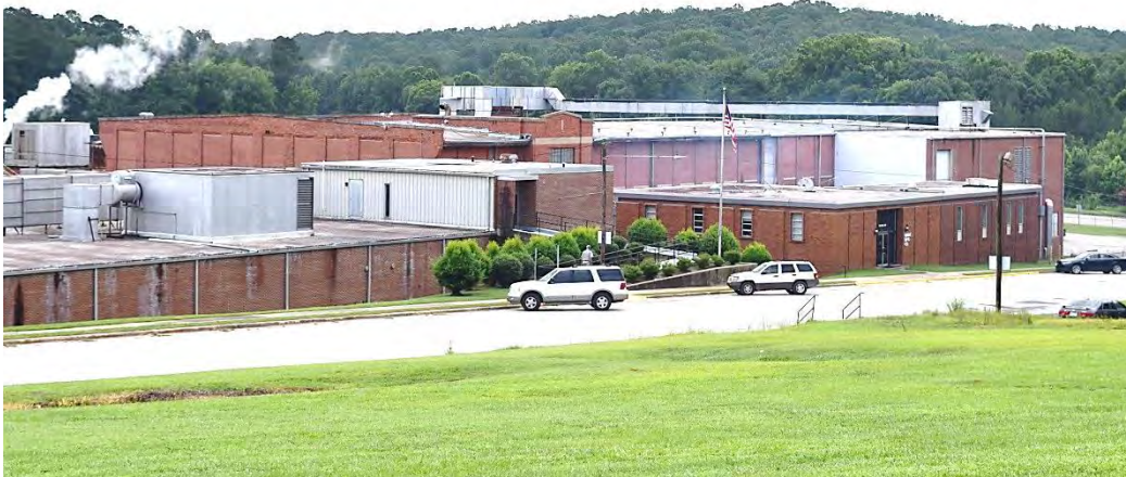
Wade Manufacturing Company and Mill Village Historic District, Overall View of Mill, Looking Southeast.
