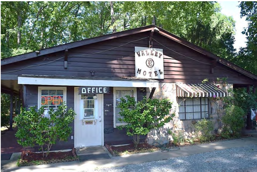
Valley Motor Court, Office Building, East Elevation, Entrance, Looking West.
