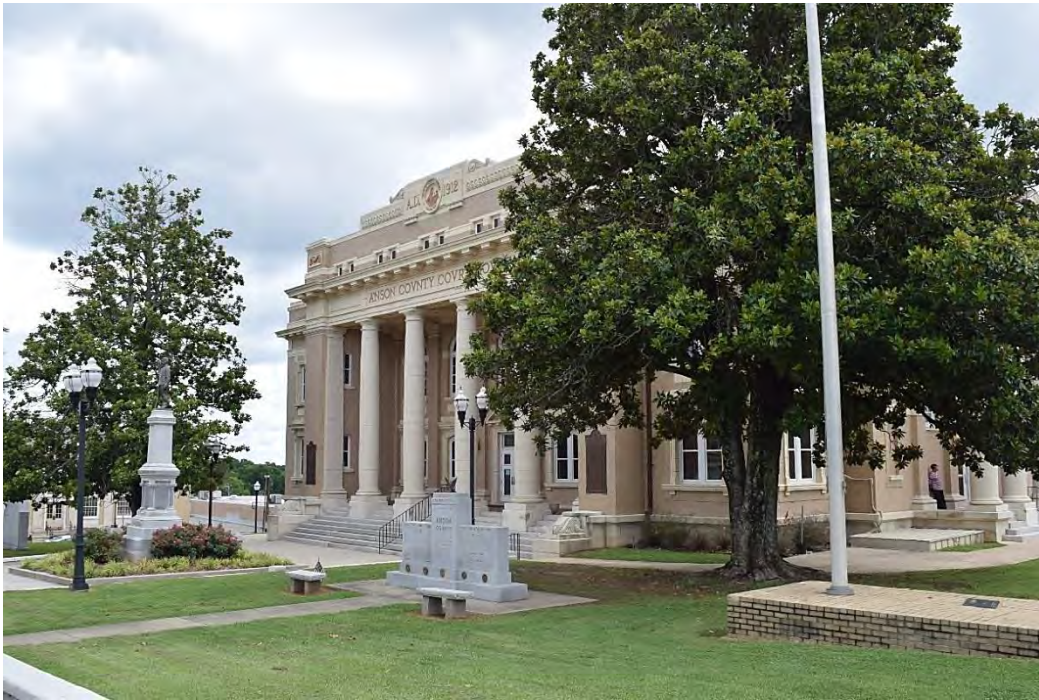
Wadesboro Downtown Historic District, Anson County Courthouse, Looking Northeast.
