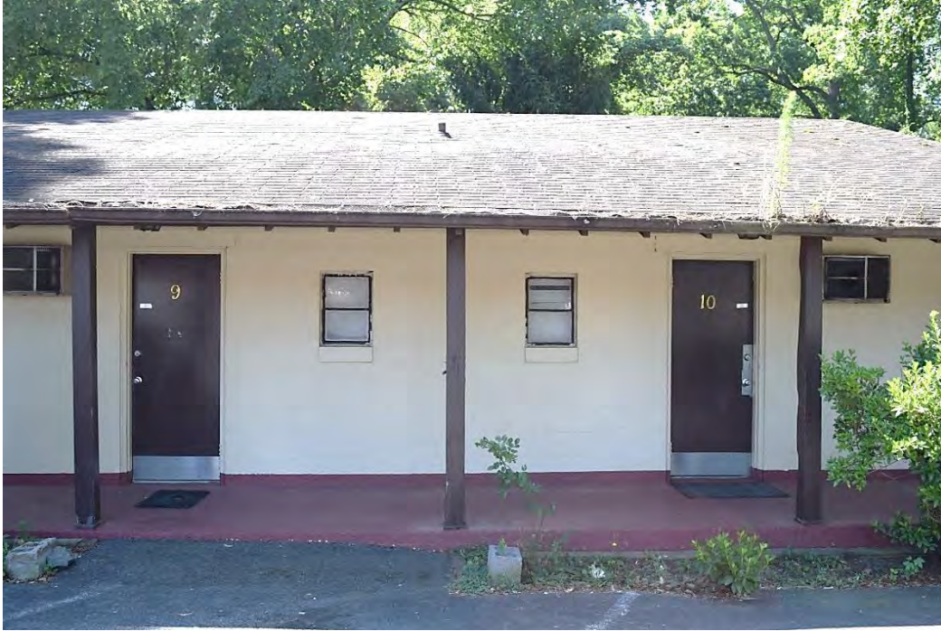
Valley Motor Court, North Building, North Elevation, Looking South.
