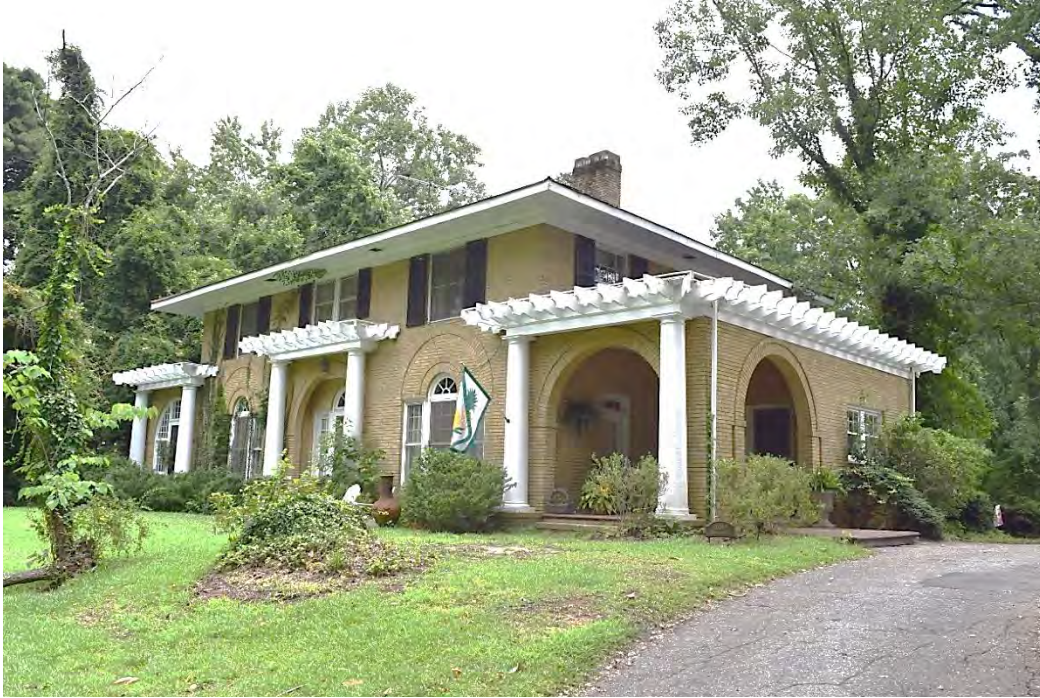
Caudle Family House, Façade (North Elevation) and Side (West) Elevation, Looking Southeast.
