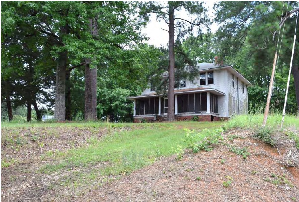
Wade Manufacturing Company Mill and Mill Village Historic District, Mill Superintendent's House, Looking North.
